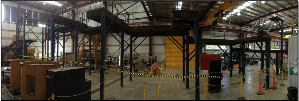
Rougher float frame assembly nearing completion. Photo taken at Gekko Systems factory in Ballarat
