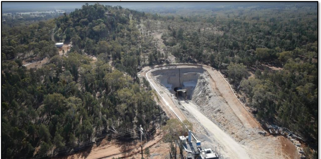
Hera Boxcut and Portal
