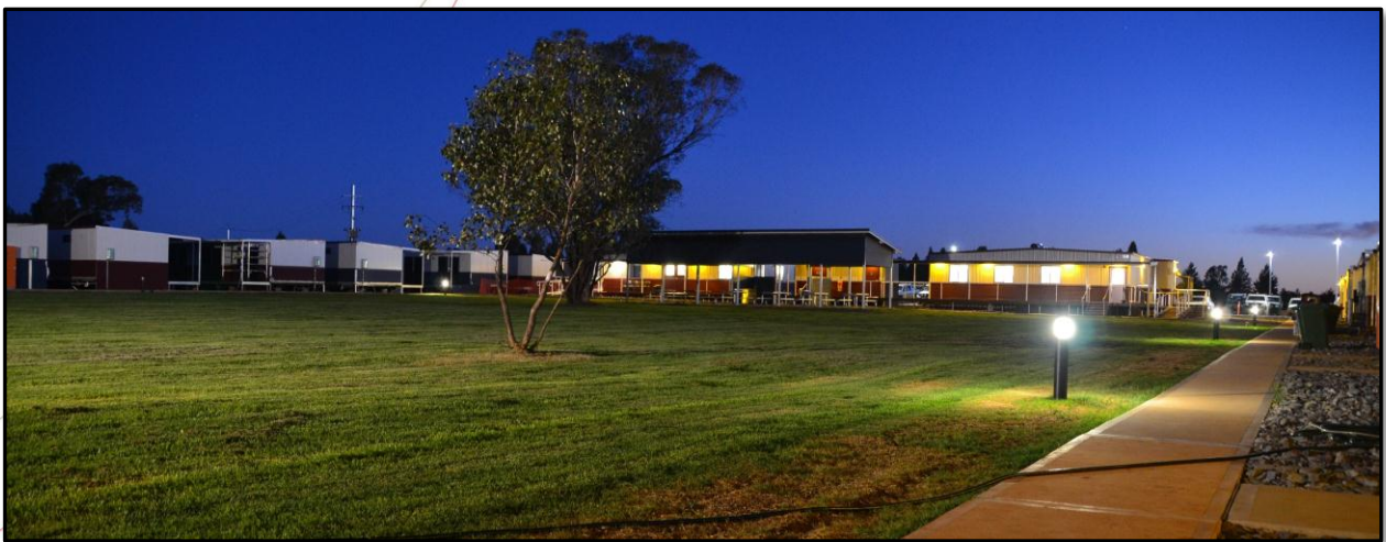
Hera Camp showing Stage 2 units under construction at left
