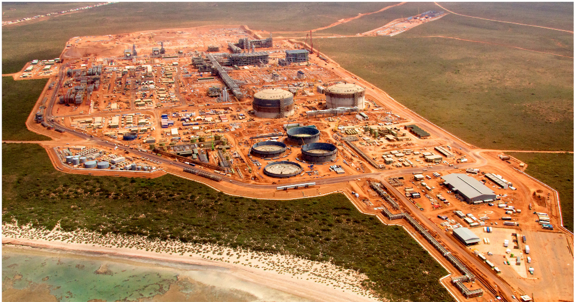
Facilities Management Services, Chevron-operated Gorgon Project, Barrow Island.
