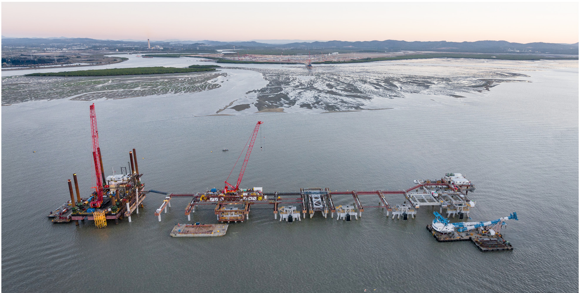
The wharf, consisting of nine modules fabricated by SinoStruct, and jack up barge at the Wiggins Island Coal Export Terminal in Gladstone, Queensland.
