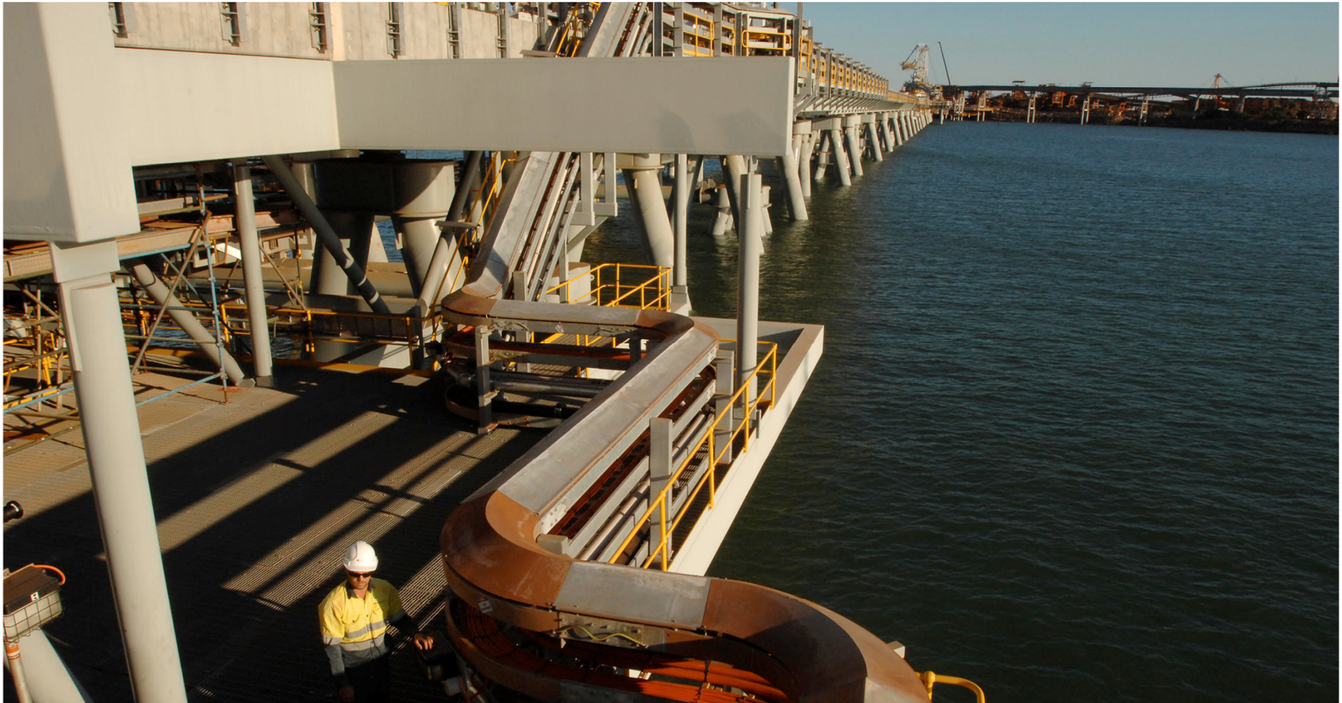
BHP Billiton Inner Harbour Project, Port Hedland.
