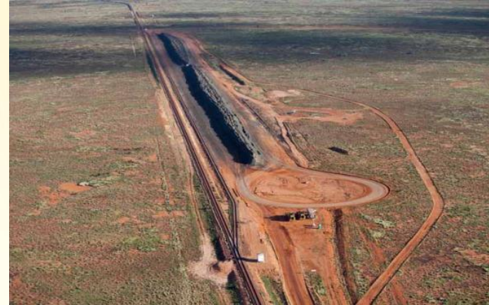
Rail Siding and Loading Facility
