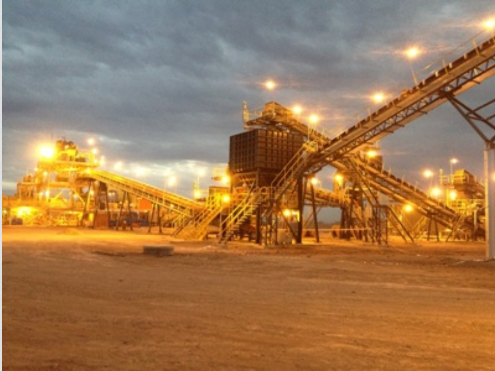
Overall plant view
