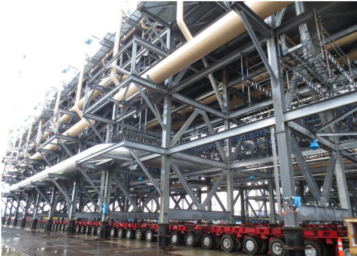
Propane condenser module ready for load-out in the Philippines
