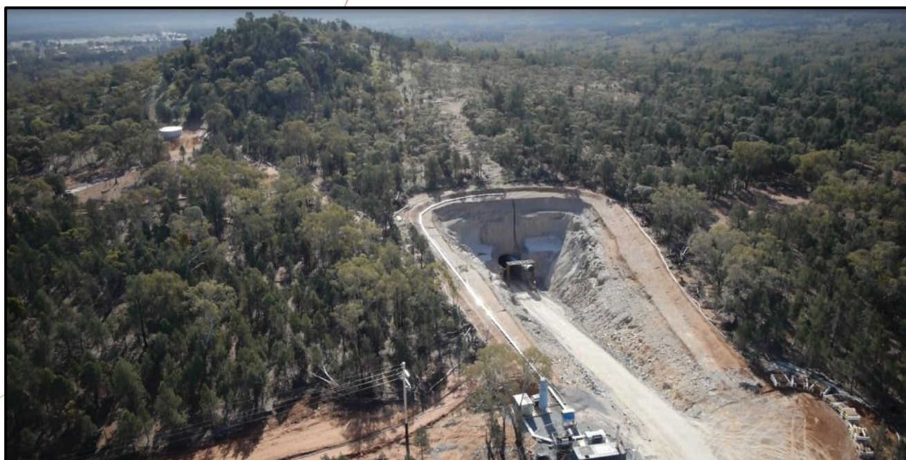
Hera Boxcut and Portal
