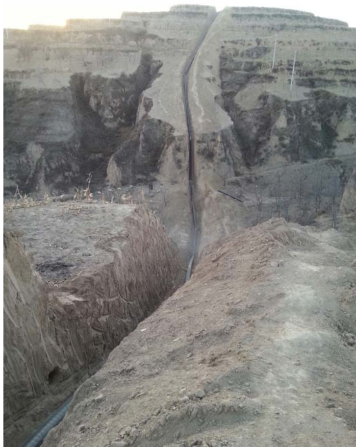
Construction of the third-party spur pipeline commenced
