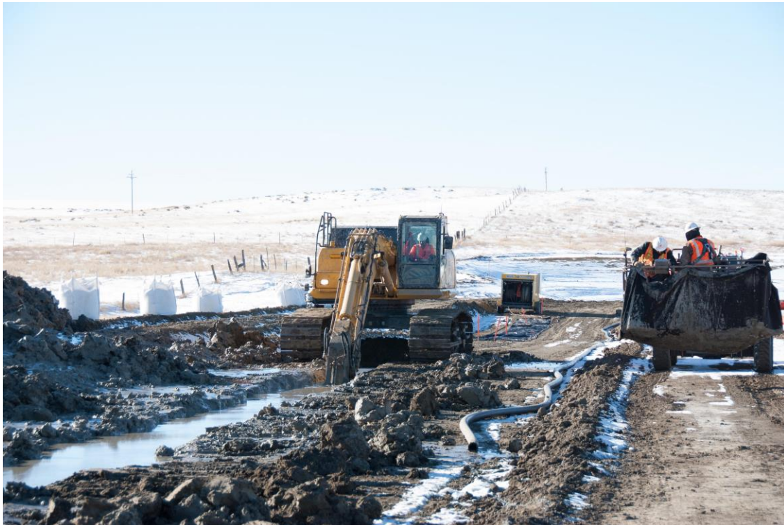
Figure 1: Containment Barrier Wall at Ross Permit Area, Wyoming USA
