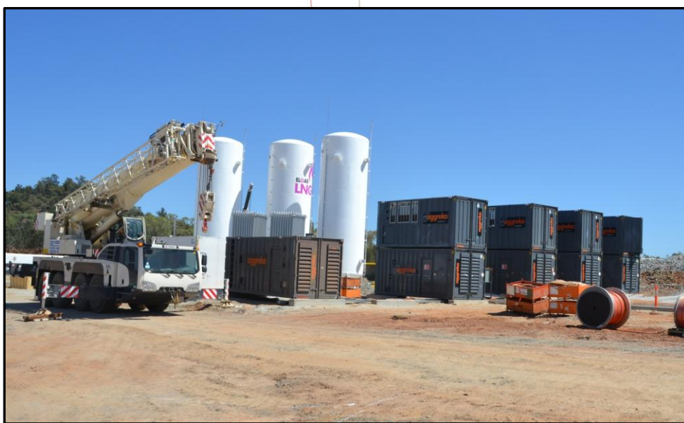
Construction of the Hera power station
