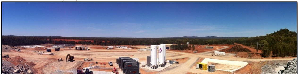
Panorama of Hera Project Construction Site
