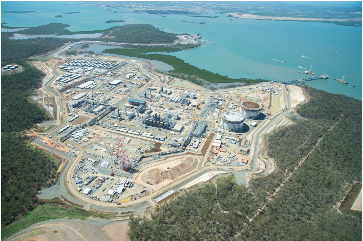
GLNG plant site on Curtis Island, 2 December 2013.
