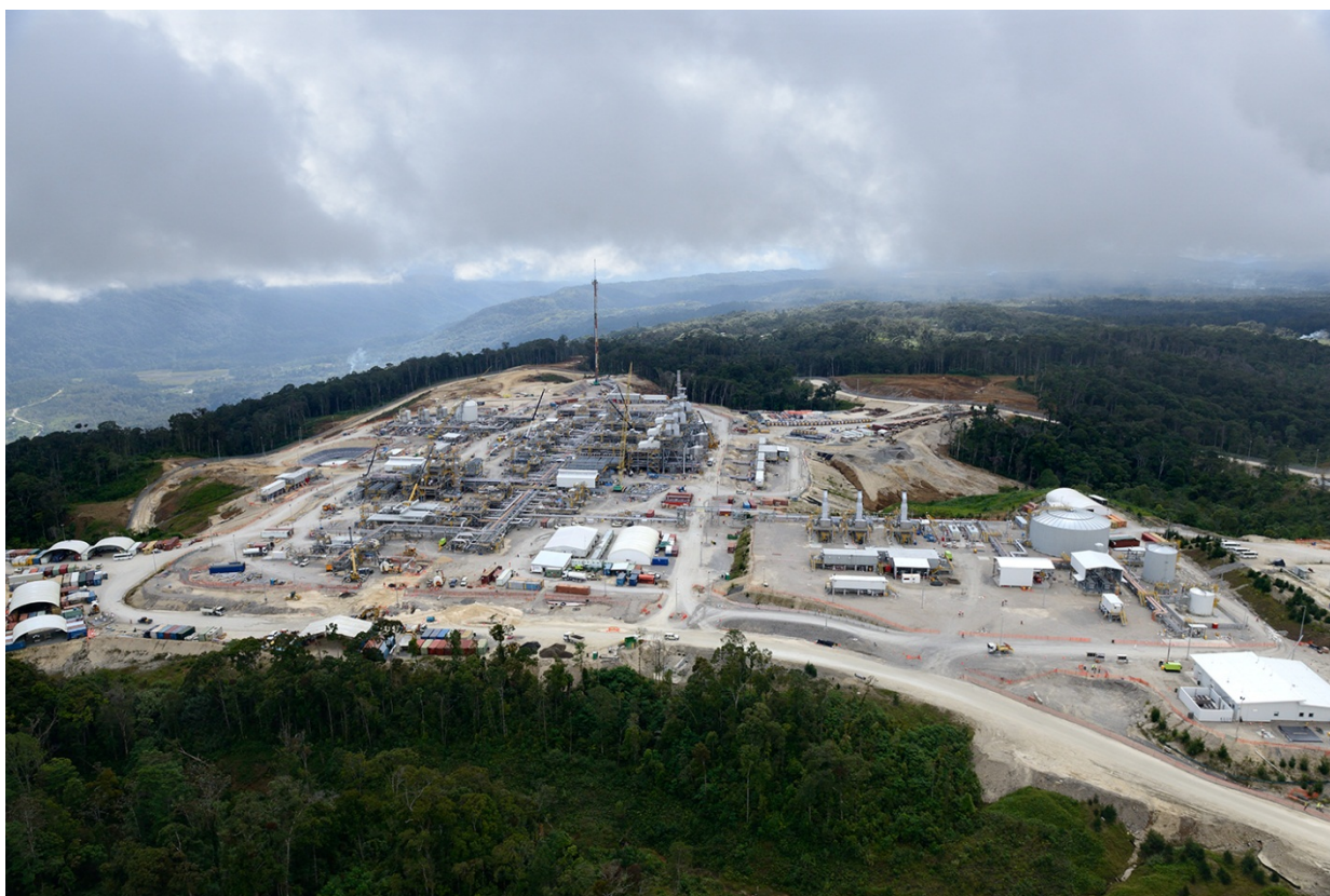
Hides Gas Conditioning Plant, PNG LNG, November 2013.
