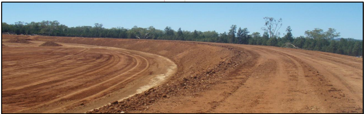
Completed TSF wall
