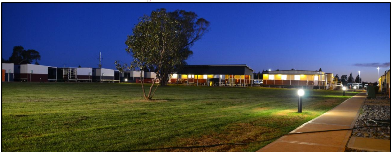
Hera Accommodation Camp
