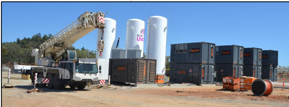
Construction of the Hera power station
