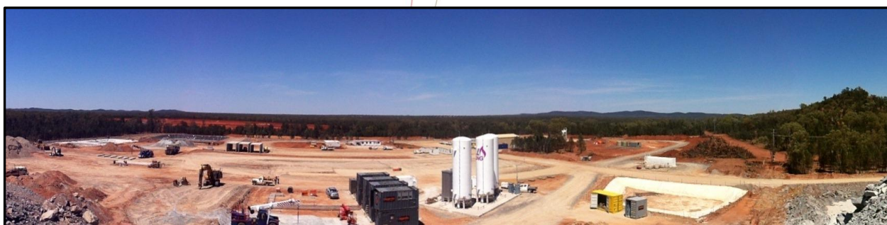
Panorama of Hera Project Construction Site
