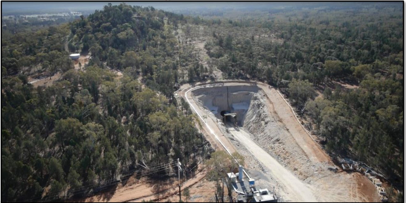
Hera Boxcut and Portal
