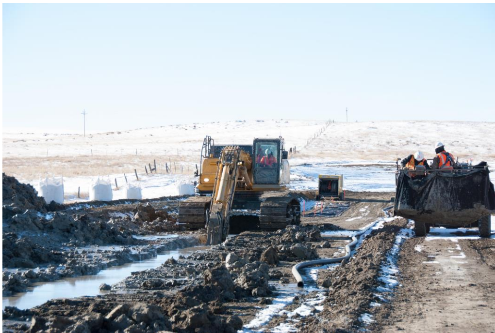
Figure 4: Containment Barrier Wall at Ross Permit Area, Wyoming USA
