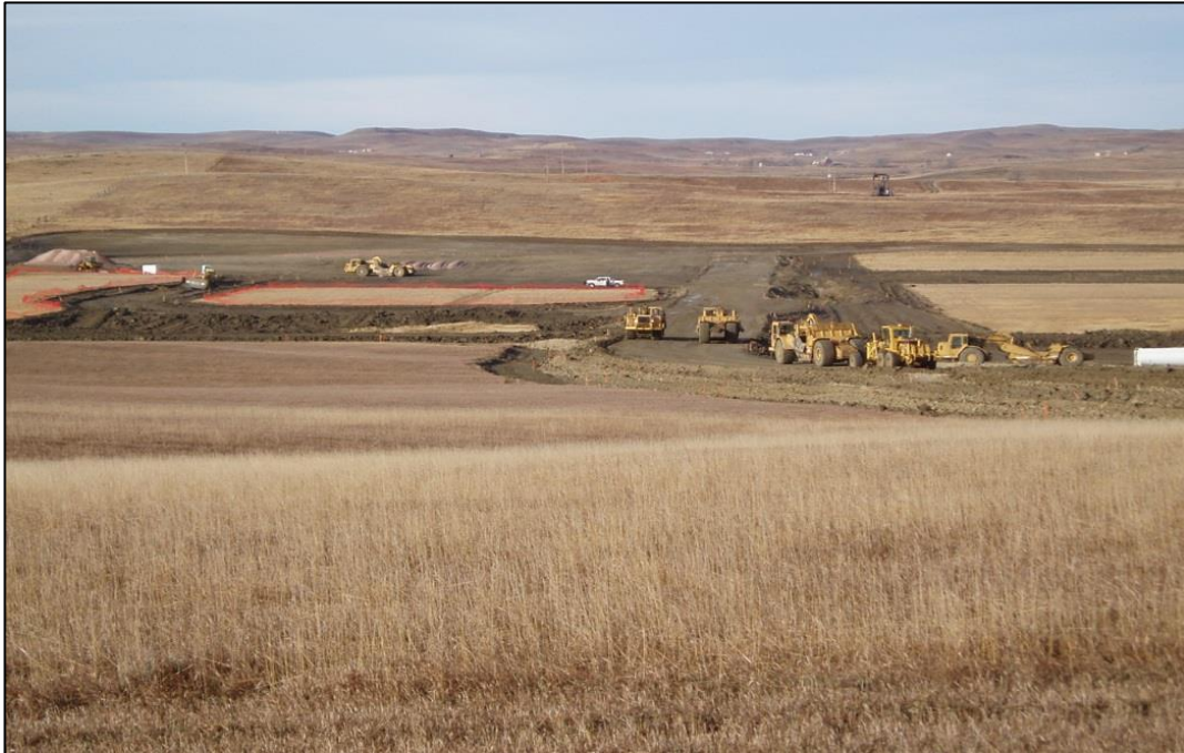
Figure 2: Earthworks at Ross Permit Area, Wyoming USA
