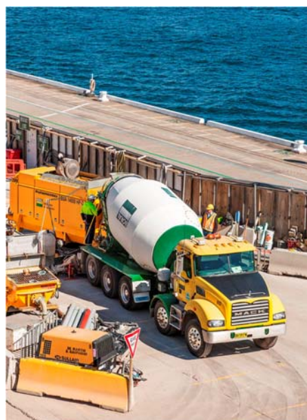
Delivering concrete to Barangaroo project
