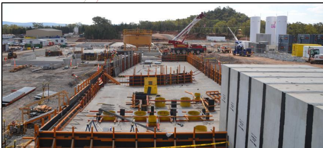
Recent photo of Hera process plant site. Tertiary crusher footings are shown in the foreground, leach feed thickening tank (yellow) in the centre and power station at right
