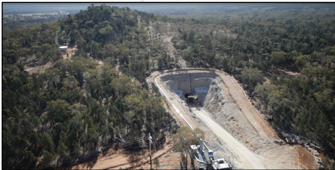
Hera Boxcut and Portal
