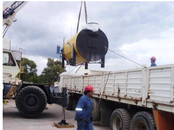
Boiler being loaded for relocation
