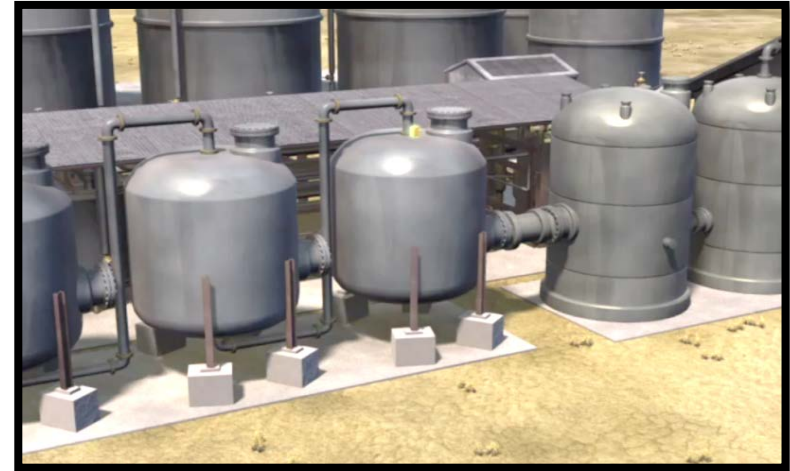
Central Processing Plant: Ion Exchange Vessels (left), Elution circuit (right)
