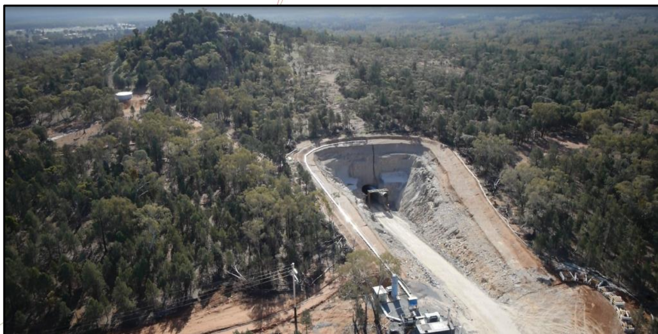
Hera Boxcut and Portal
