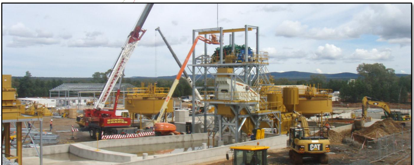
Recent photo of construction at the Hera process plant site.
