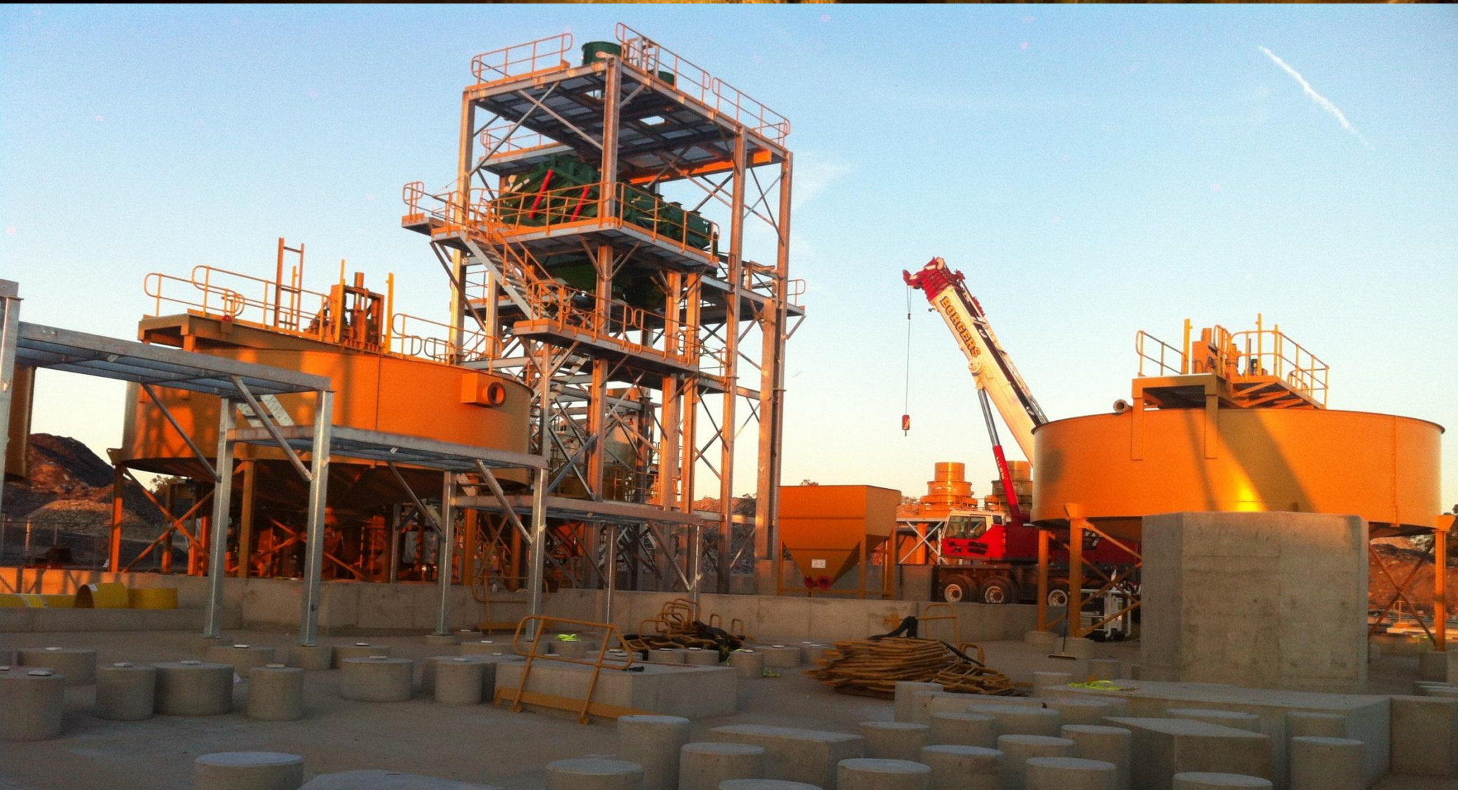
Hera Mill Construction
