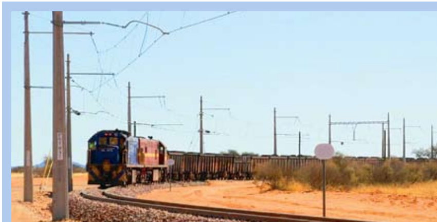
Tshipi Rail Siding
