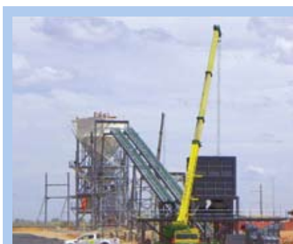
Construction of the rapid load out station and feed conveyors
