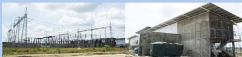
Substation Control Building
