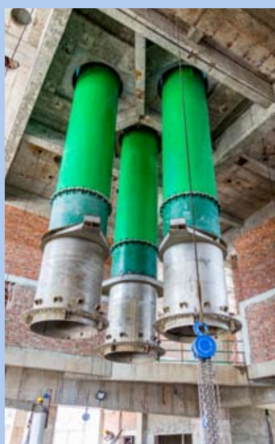
A01 workshop furnace electrode holder erection and welding
