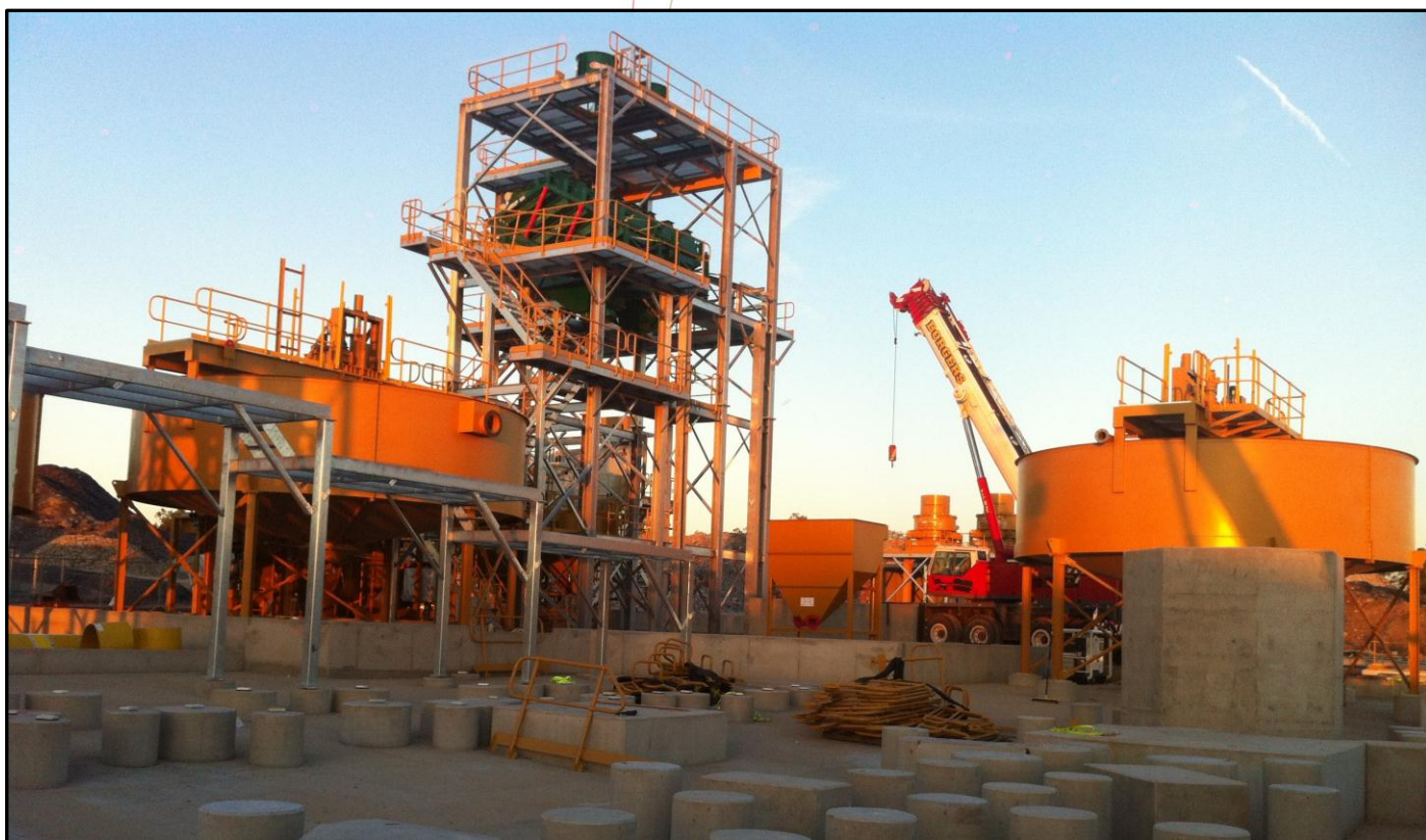
Process Plant construction – 31 st March, gravity frame at centre.
