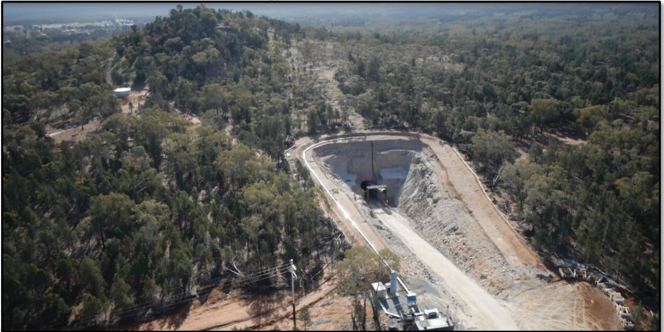
Hera Boxcut and Portal
