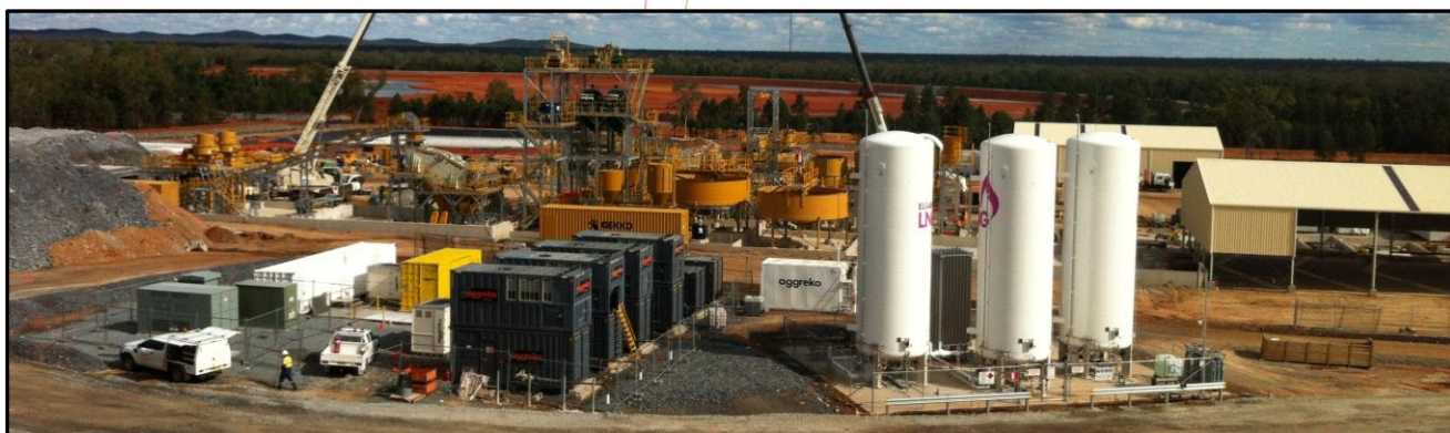
Hera Project Construction – April 2014
