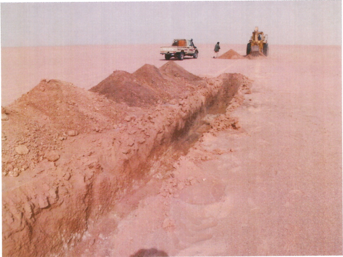
Figure 4; Trench showing pale calcrete mineralisation under a thin cover of wind-blown sand
