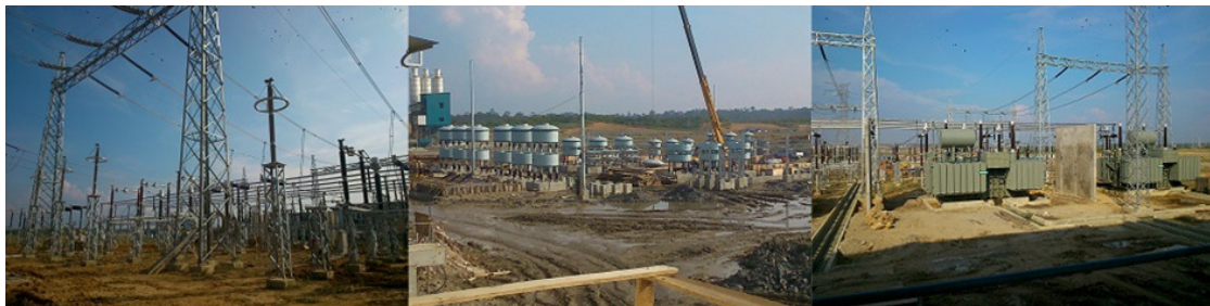
Substation Control Building
