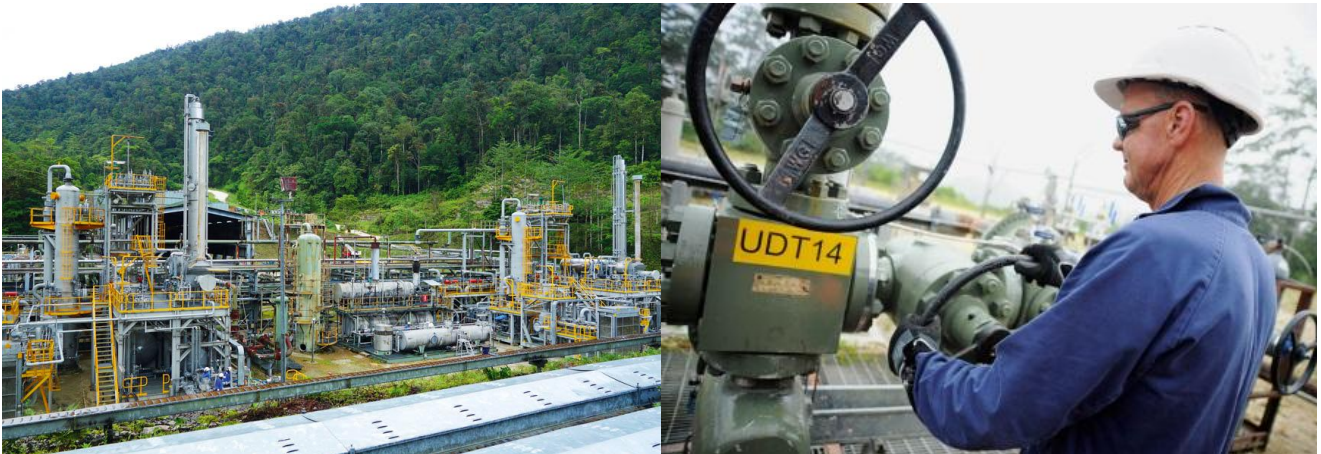
Central Processing Facility, Kutubu
