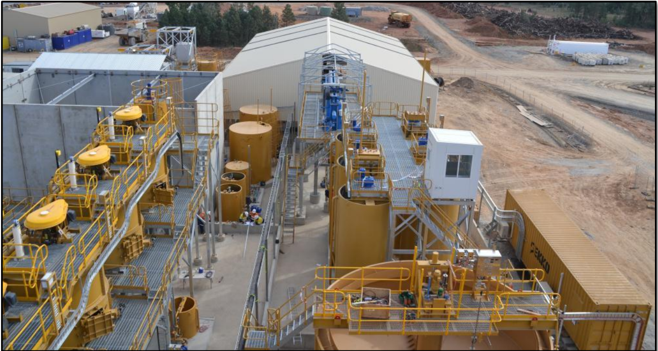
Hera Process Plant construction: Rougher flotation cells at left, leach tanks in middle ground and concentrate storage shed at rear
