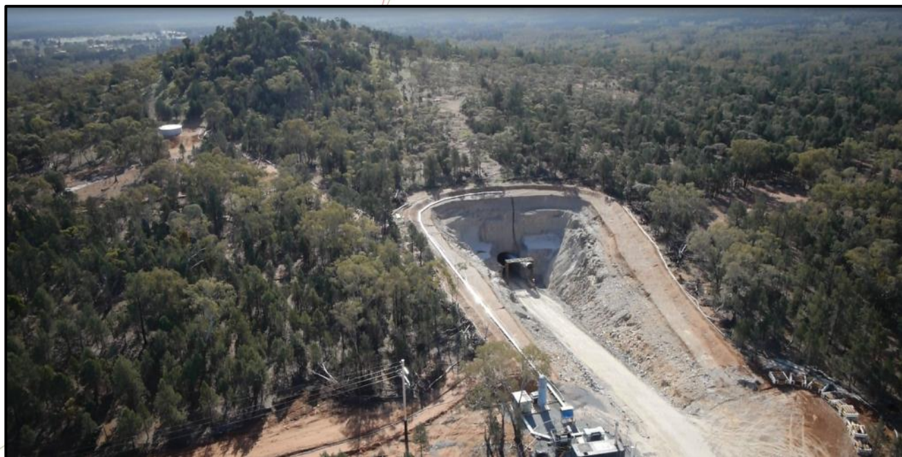
Hera Boxcut and Portal
