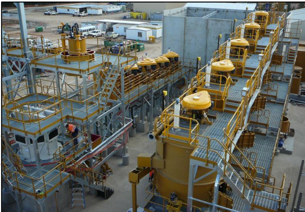
Hera Process Plant construction: Re-grind mill at left, cleaner flotation cells in middle ground and rougher flotation cells at right
