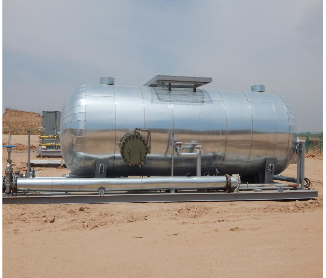
Separator at Sanjiaobei Central Gathering Station
