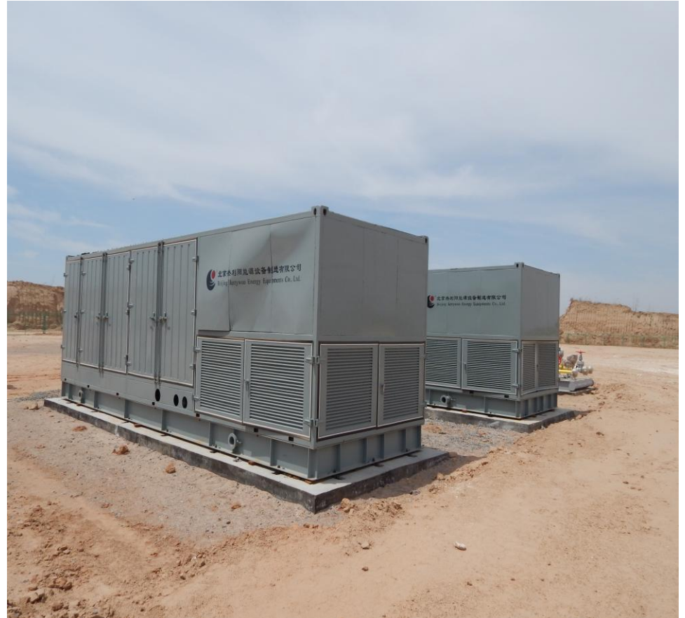
Gas Compressors at the Sanjiaobei Central Gathering Station
