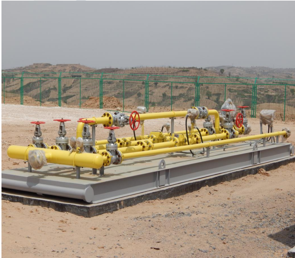
Flow metre station at Sanjiaobei
