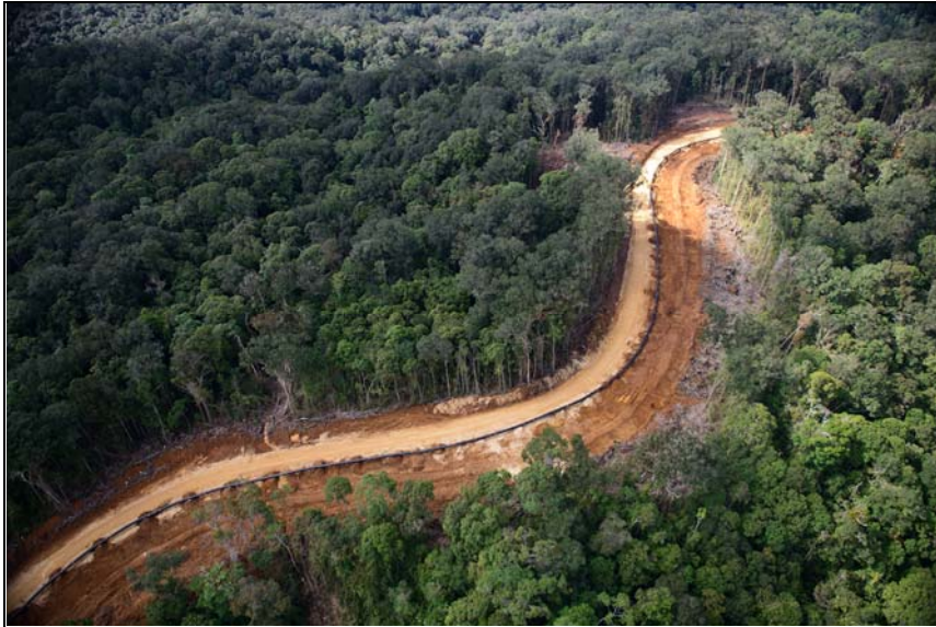
Onshore pipeline at Hides November 2013
