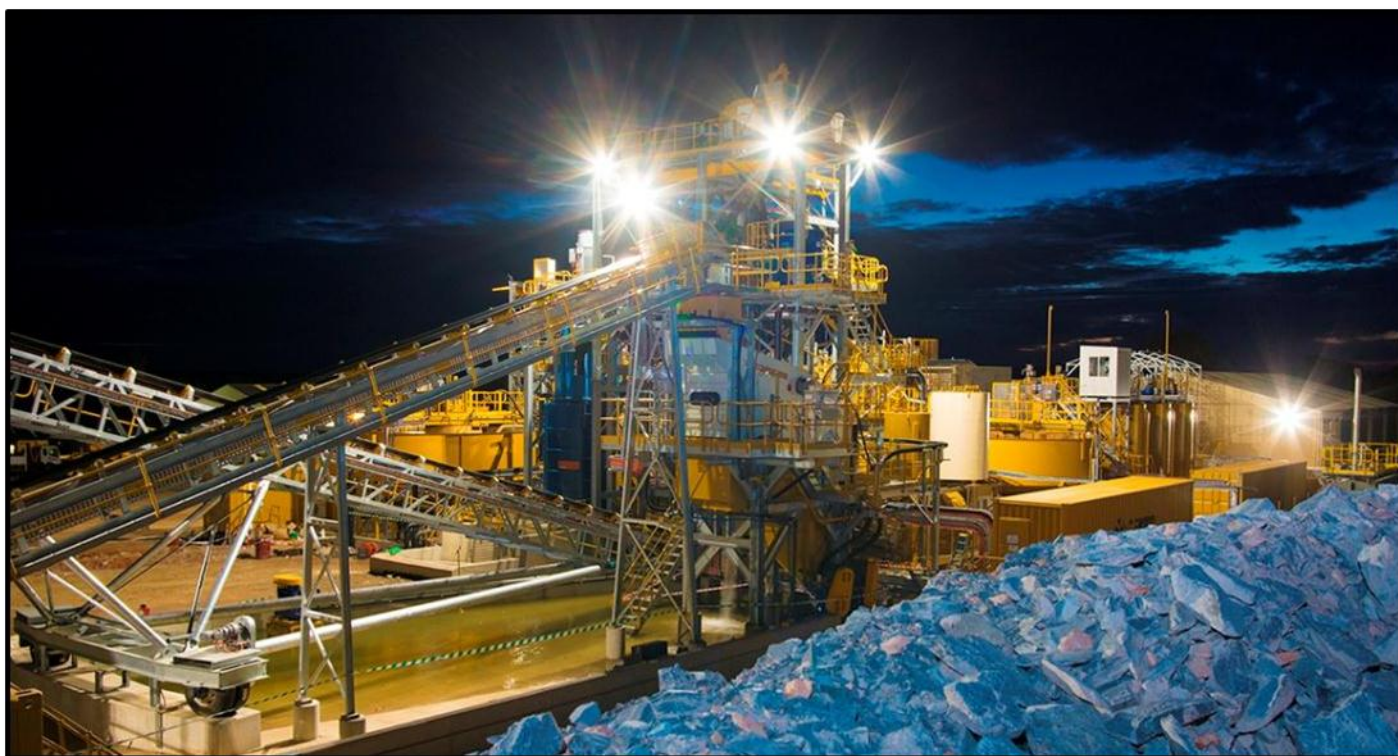
Hera Processing Plant
