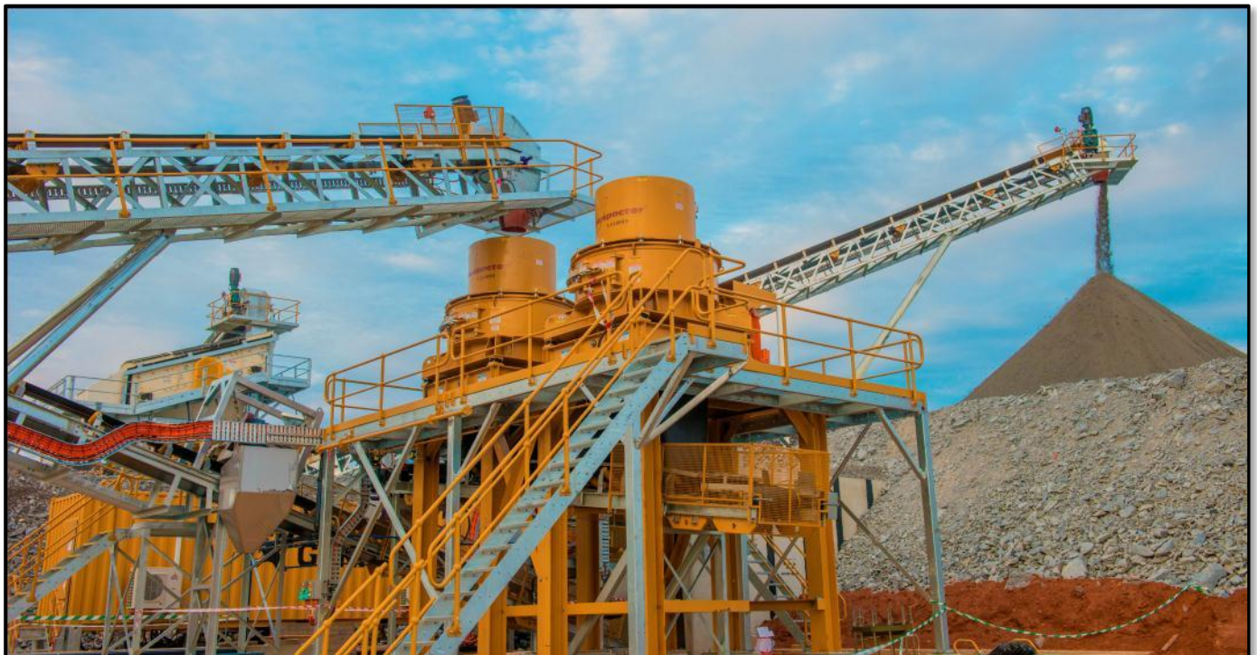
Crushing circuit under commissioning
