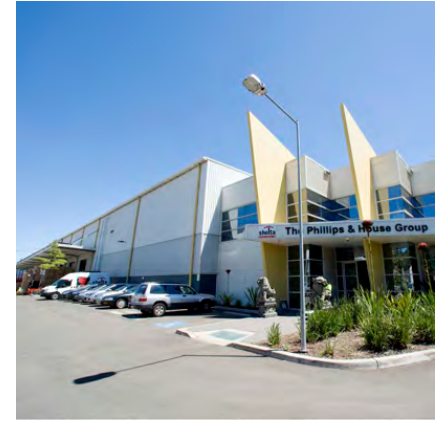
1 Foundation Place, Greystanes
