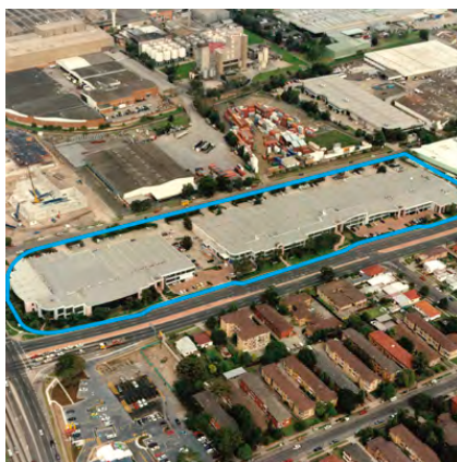
79-99 St Hilliers Road, Auburn
