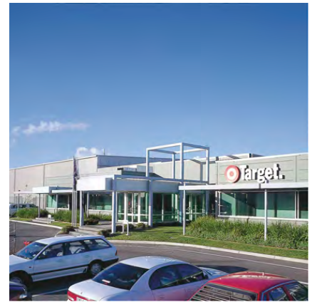
Target Distribution Centre, 30-68 Taxis Avenue, Altona North
