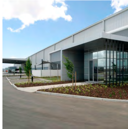
DEXUS Industrial Estate, 1 Foundation Road, Laverton North
