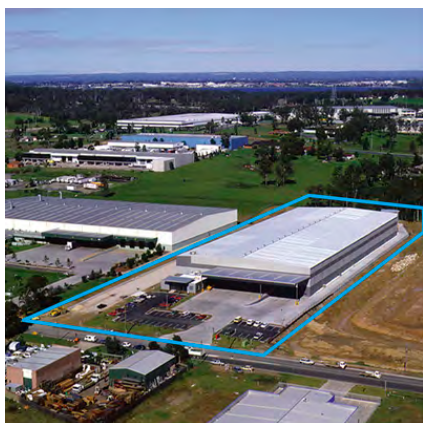
52 Holbeche Road, Arndell Park
