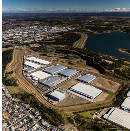
Quarry Industrial Estate, Reconciliation Road, Greystanes
