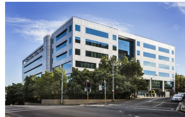
12-22 Woniara Road, Hurstville, NSW - exterior
