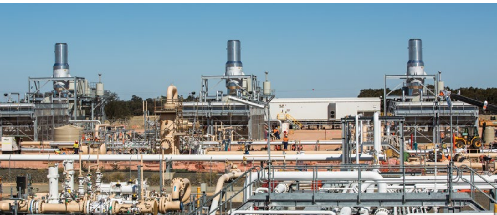
Three new Solar Mars 90 compressors installed at Wallumbilla, adding to six existing compressor units.
