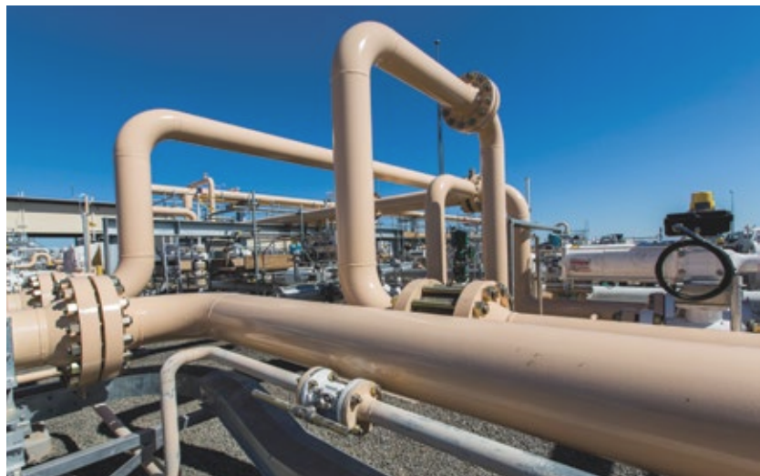
Modification of the SWQP pipeline at Wallumbilla to allow bi-directional flow capability.
