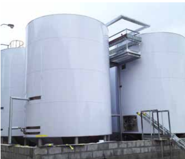
Stage 3: Insulation of tallow tanks
