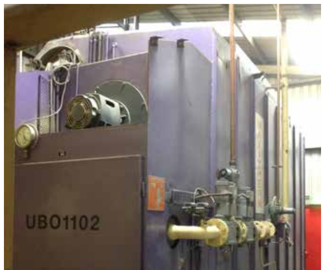
Stage 4: Boiler upgrade
