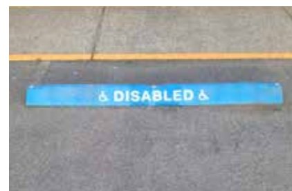
Wheel stops at new Pakenham car park made from Ridley's plastic waste.
