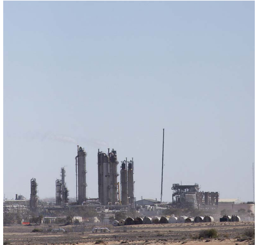
The key processing point for Cooper Basin and Eromanga Basin oil and raw gas
