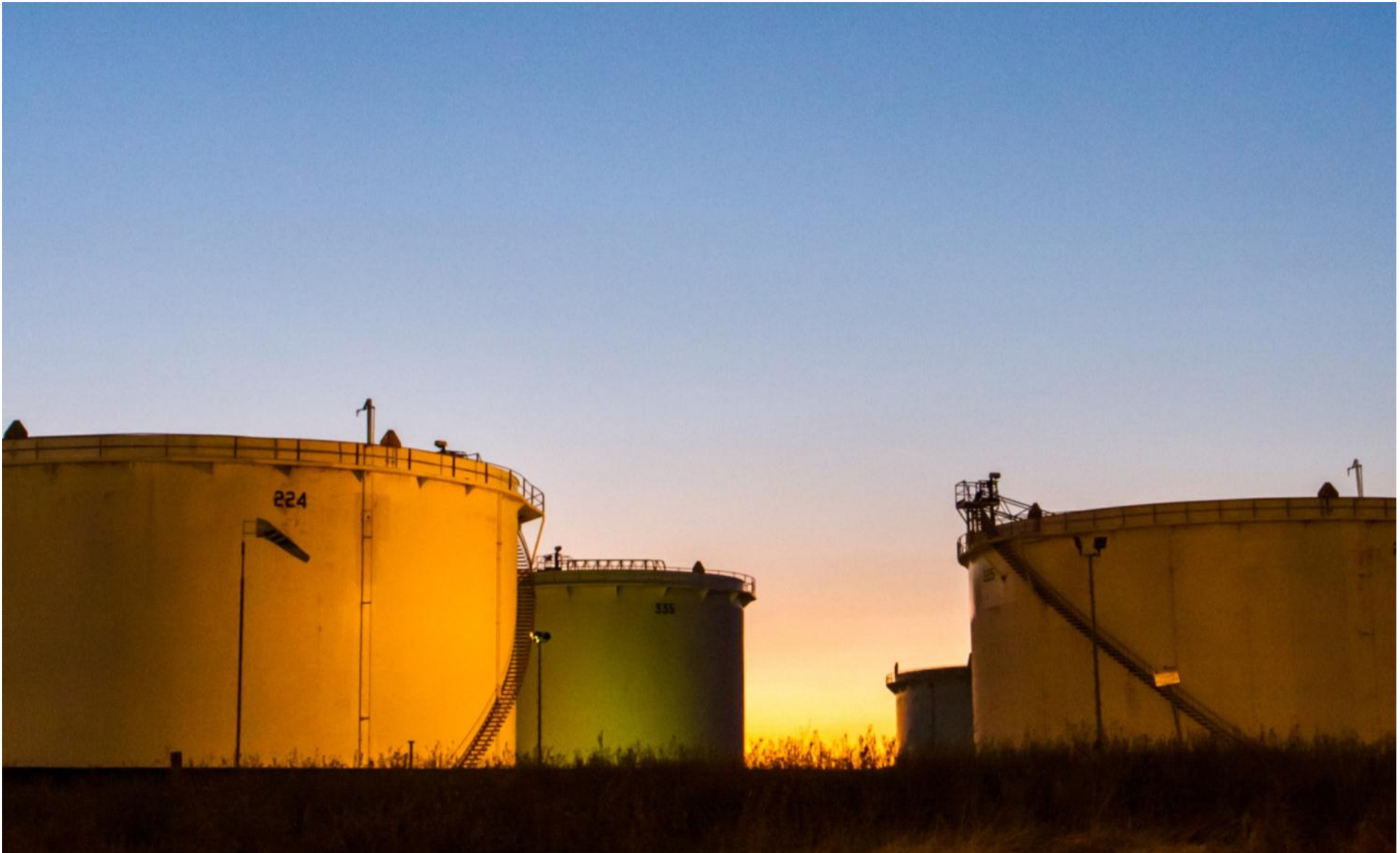
Product tanks at Kurnell Refinery
