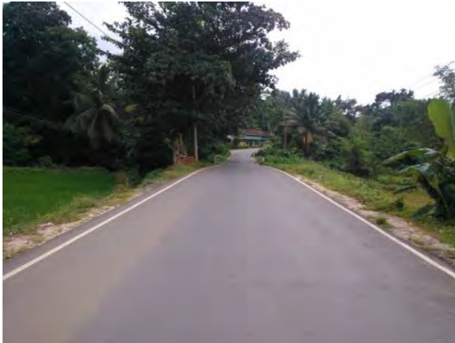
Figure 9: Primary Tar Road Close to EL237 Area
