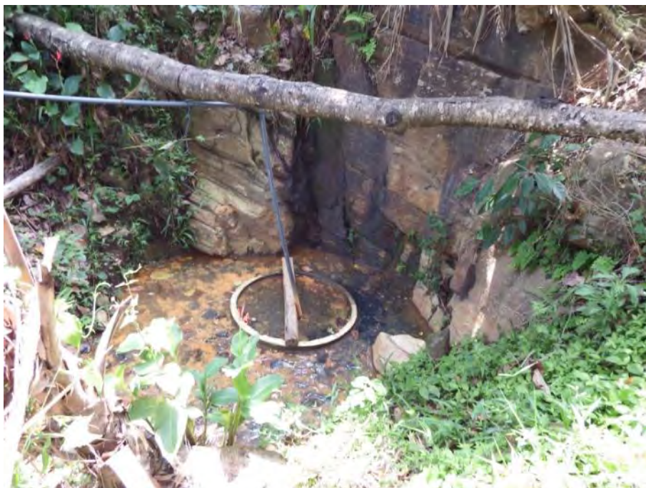
Figure 24: Flooded declined adit in EL953
