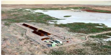
The highly automated stockyard, with a stacker and reclaimer, will load the TSV via the conveyor
