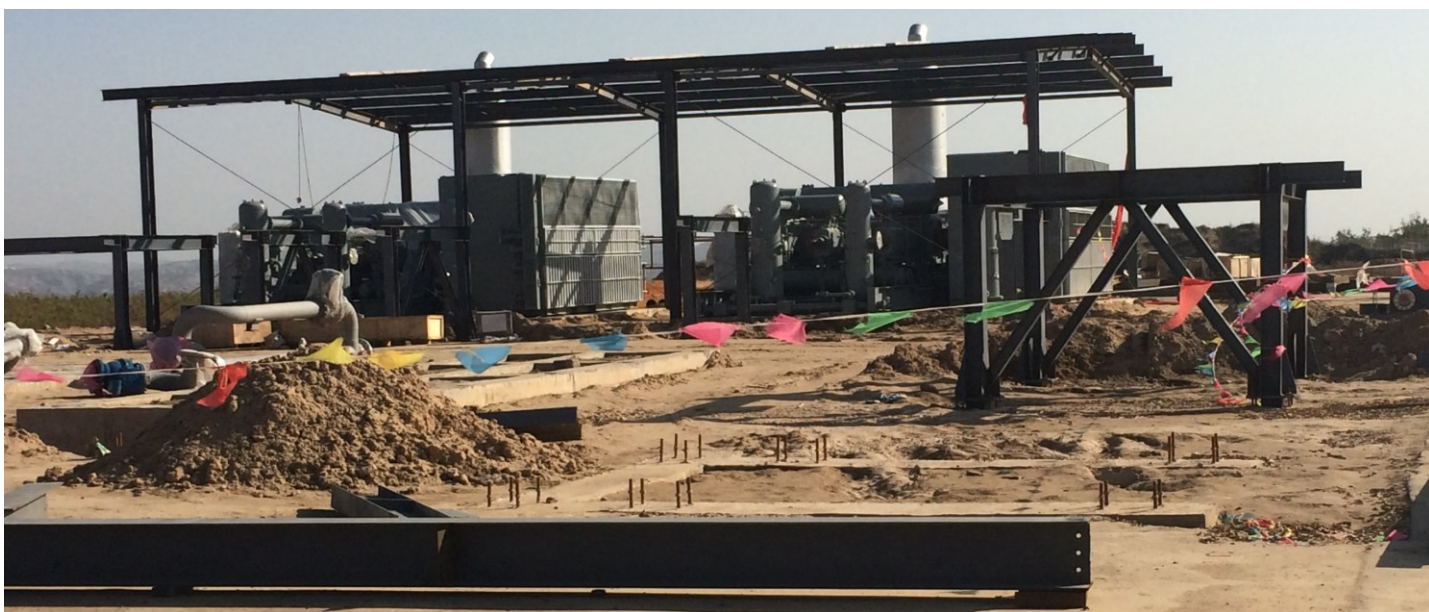
Installation and connection of the production equipment on the Linxing central gathering station
