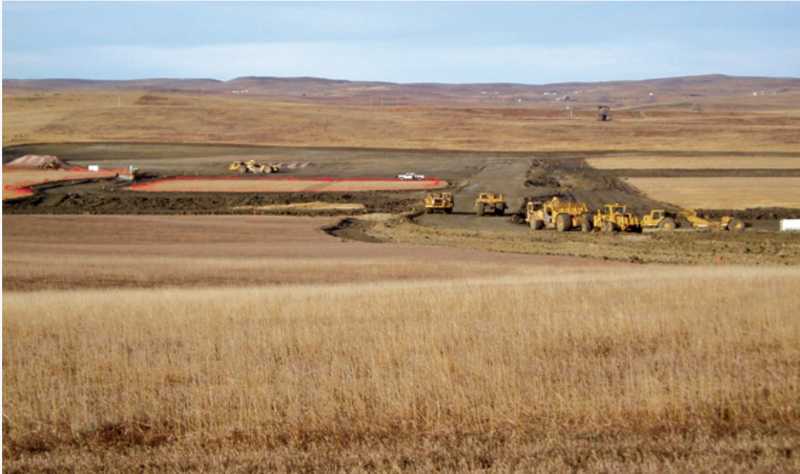
Figure 2: Earthworks for the CPP, November 2013, Wyoming, USA
