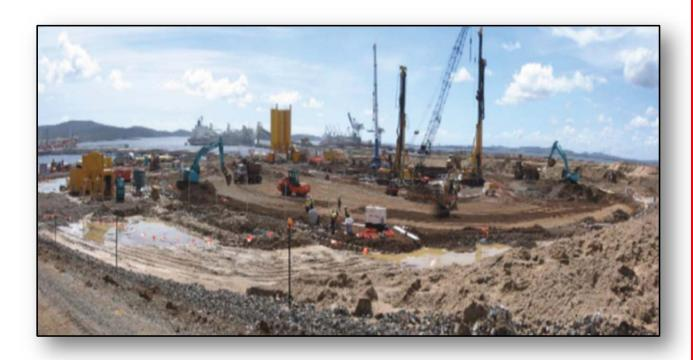
**Figure 2:** Site Construction at Fisherman's Landing (March 2010) showing Earthworks and Tank Piling Deep Soil Mixing
