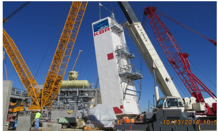
Ammonia tank refrigeration equipment under construction
