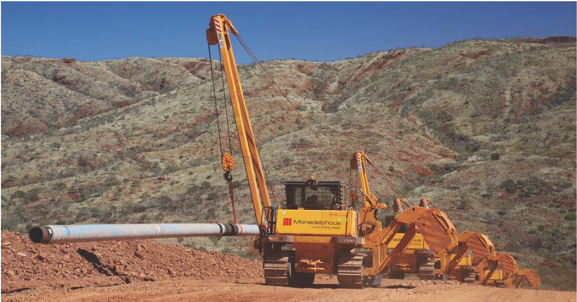
Rio Tinto West Angelas Gas Pipeline, Newman, WA
