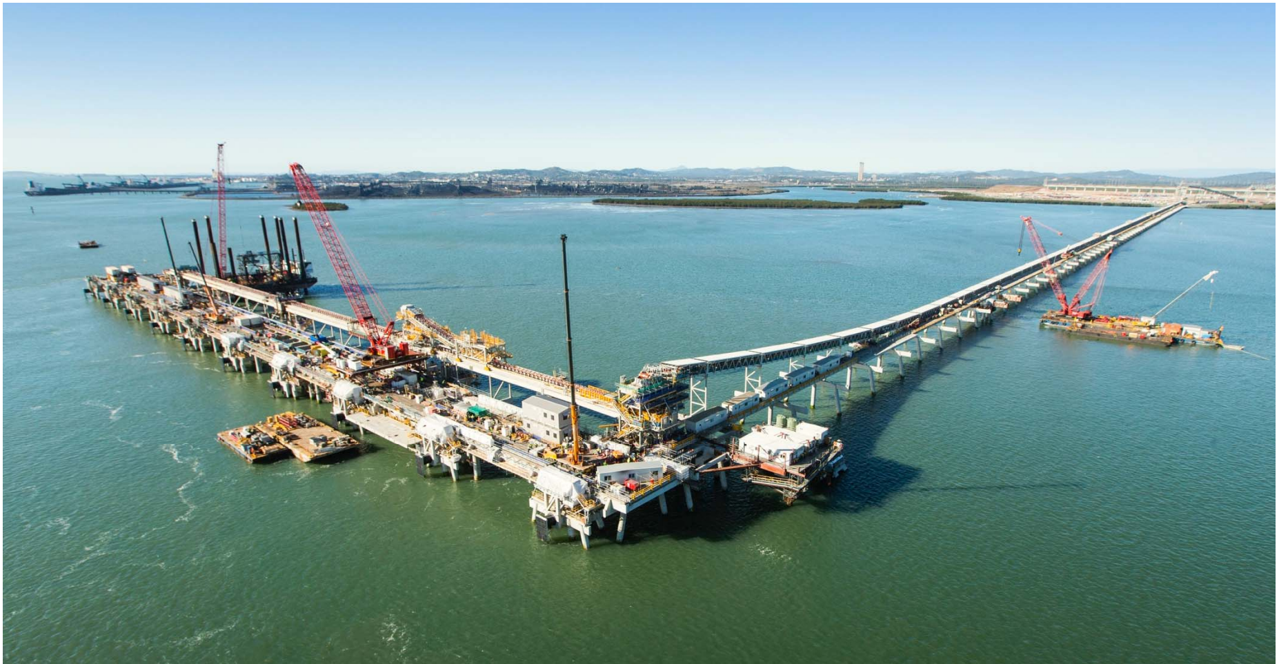
Wiggins Island Coal Export Terminal, Gladstone, Queensland
