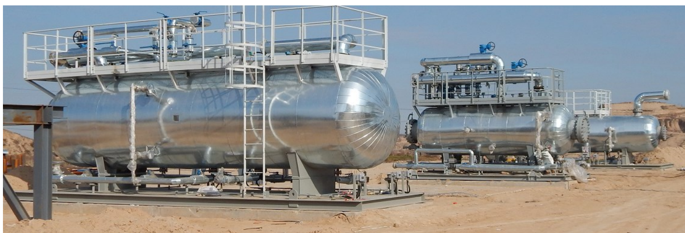
Installation and connection of separators on the Linxing central gathering station
