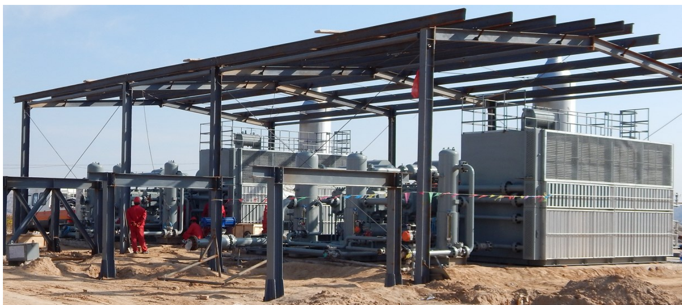
Installation and connection of compressors on the Linxing central gathering station
