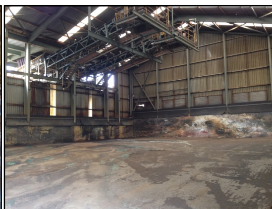
Picture 4: Concentrate Storage Shed & Bagging Station
