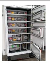
Where there in inadequate room in a MSC isolator cubicle for the remote isolation hardware, REMSAFE install a Failsafe Instrument Cubicle nearby
