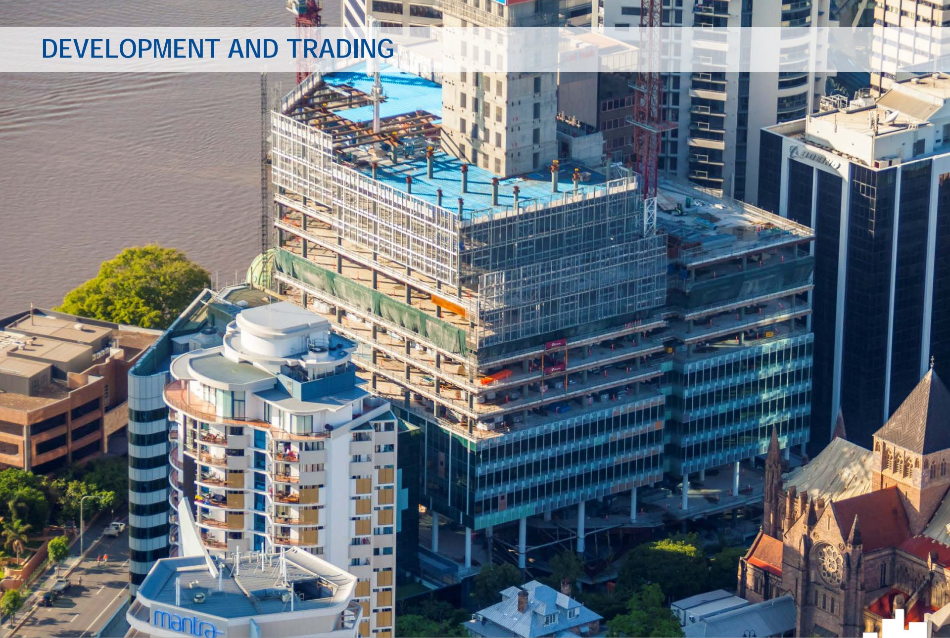
480 Queen Street, Brisbane QLD (under construction).
