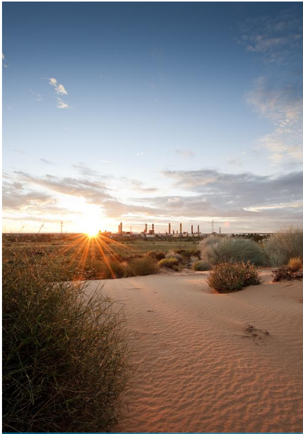
Moomba Plant, Cooper Basin
