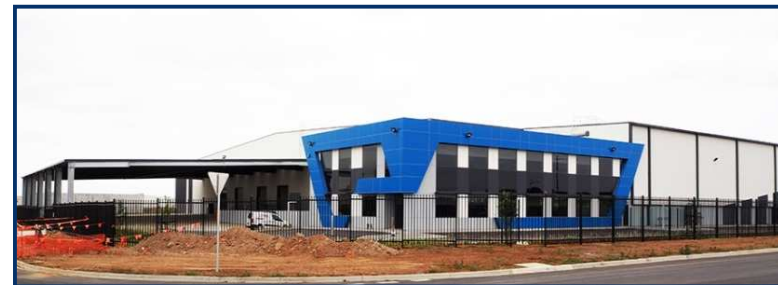
New Warehouse near Completion
