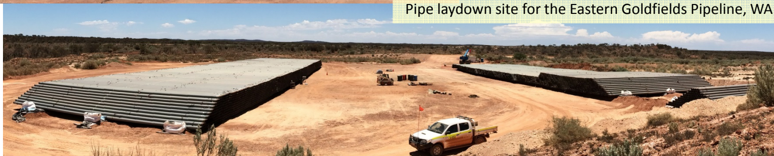
Pipe laydown site for the Eastern Goldfields Pipeline, WA
