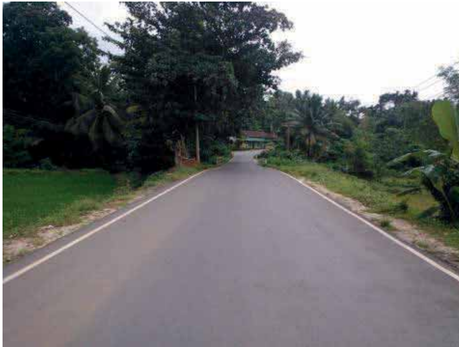
Figure 9: Primary Tar Road Close to EL237 Area
