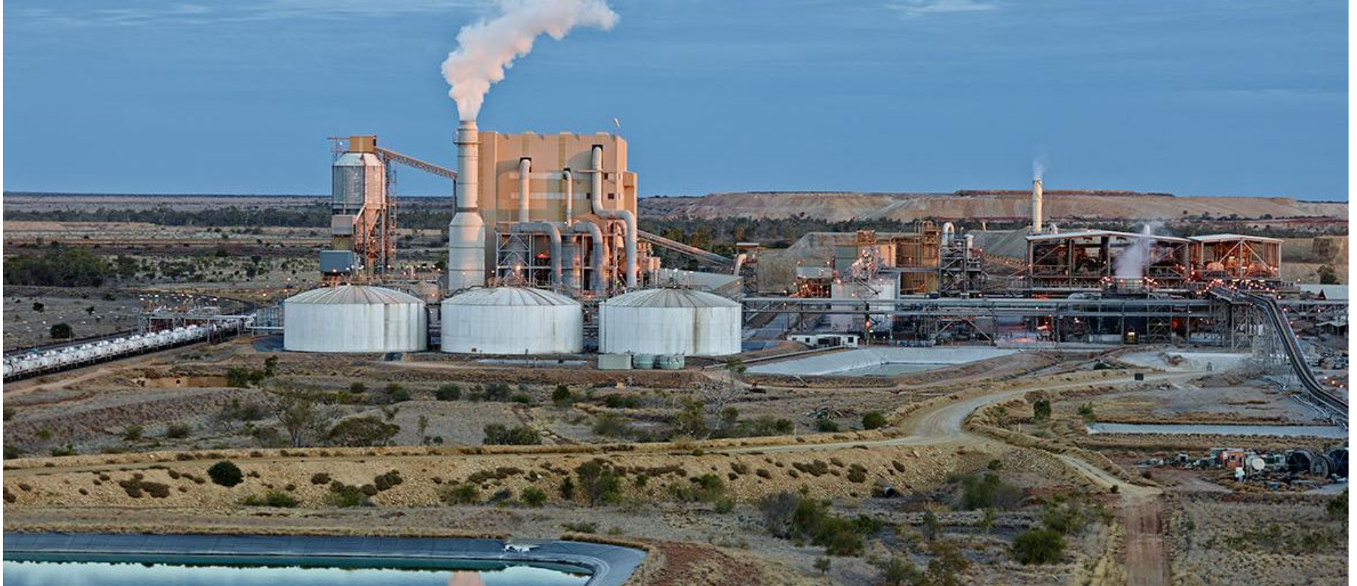
Picture: Phosphate Hill manufacturing facility, Qld, Australia
