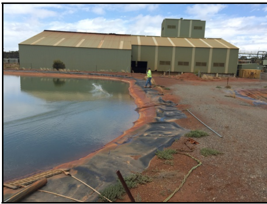
Picture 1: Process Water Dam & Concentrate Storage Shed
