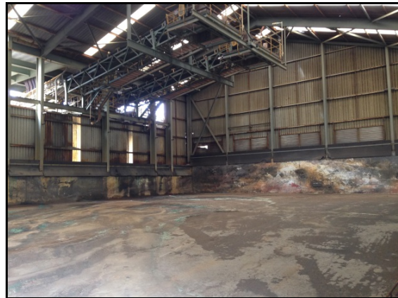
Picture 4: Concentrate Storage Shed & Bagging Station
